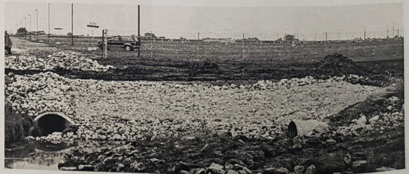
Gabion Mattress installation
