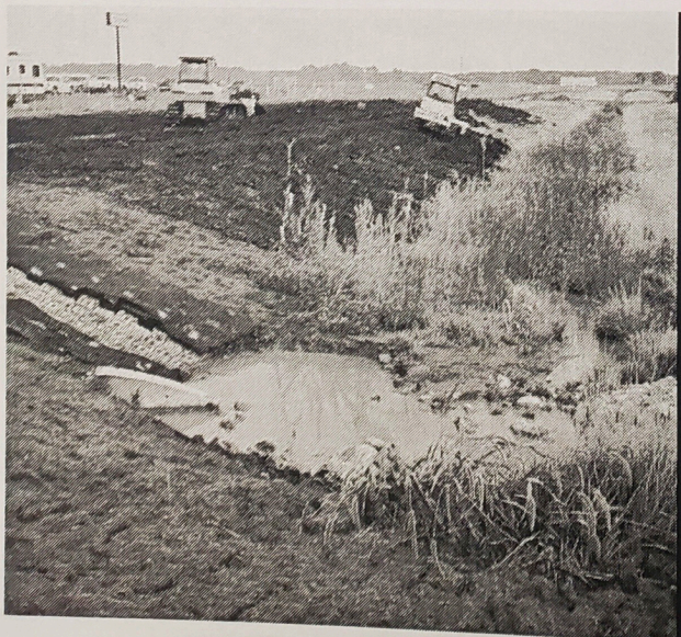
Block Chute (above) Armor Lock block and hydro-seeding (below)
