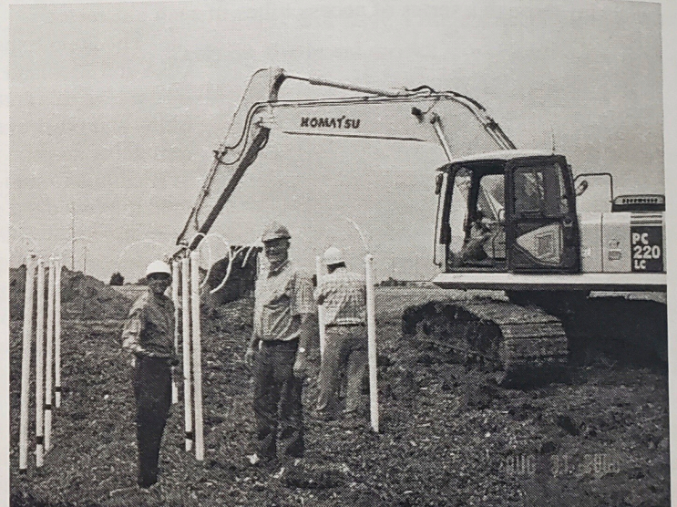
Water quality testing access tubes throughout experimental Bioreactor (above)
